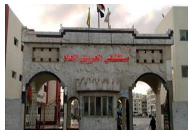
Electromechanical works for the development of Al-Arish General Hospital
