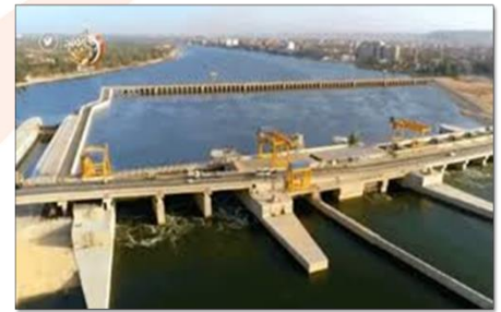
Development of the Assiut Barrages Supervision of the implementation of the low-voltage electrical supply network
