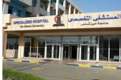
Electromechanical Works Development of the Specialized Hospital - Ain Shams University
